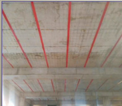
PT SLAB - RED PAINT MARKING
