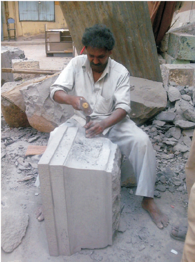
Basalt Stone Worker Carving a Stone Base for a Timber Column at Tulshibag Ram Mandir
