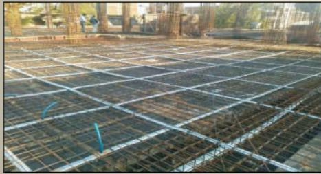
PT SLAB - LAYING
