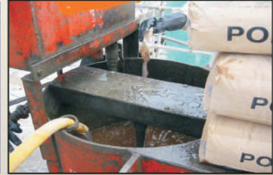
PT SLAB - GROUTING
