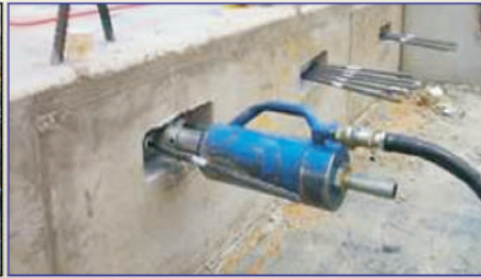
PT SLAB - STRESSING
