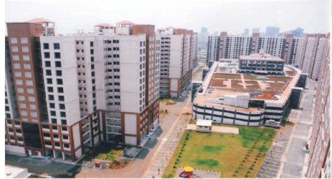
MIG & HIG Housing Project at Kharghar, Navi Mumbai for CIDCO
