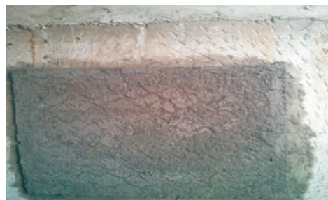
Finished Plastering on RCC wall
